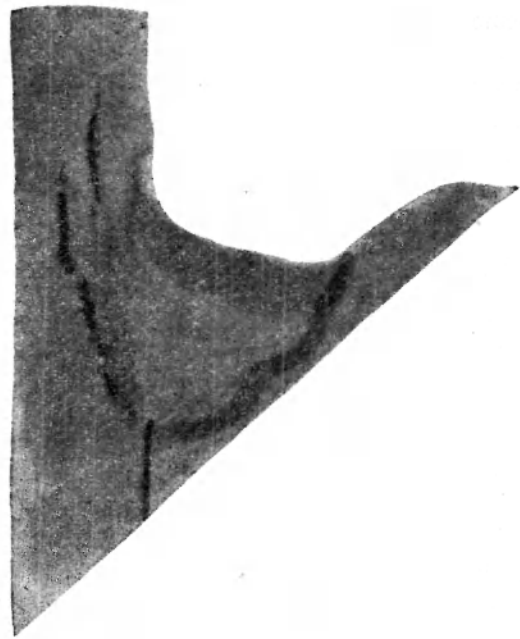
Fig. 4—Cross section of the submerged arc weld showing the rounded contour of the toe—which favoured tear resistance
