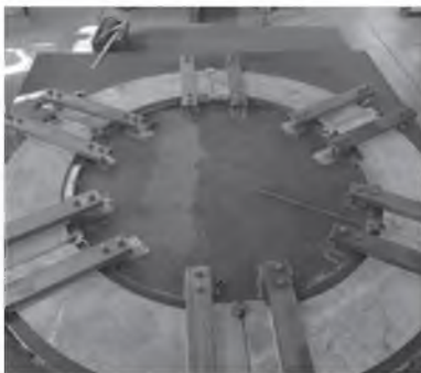
Welding using Fixtures
