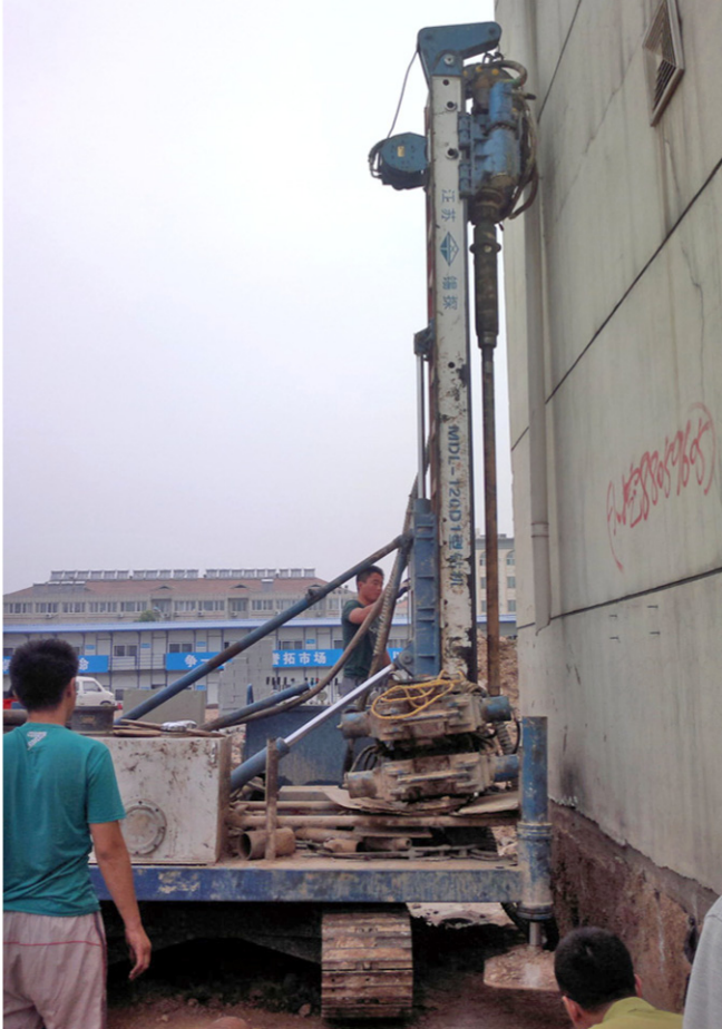
Fig.7: The drilling machine worked near the building
